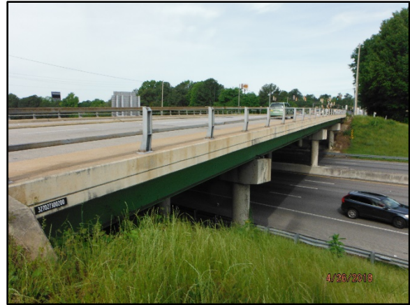
Photo 1 – S-32-273 (Bush River Rd.) Bridge over I-20 in Lexington County, SC.
